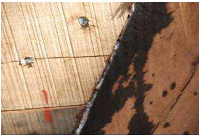
A close-up of rope caulking.
